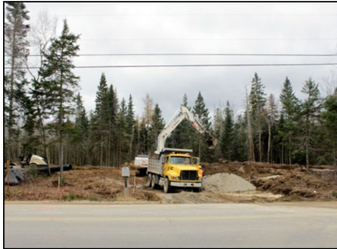
DIG IN: Crews on site in early November.
